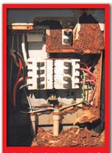
Electrical panels, unless protected will corrode due to exposure to salt air and spray, creating electrical hazards
